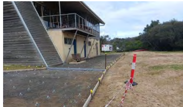
Concrete Path Works 2025
